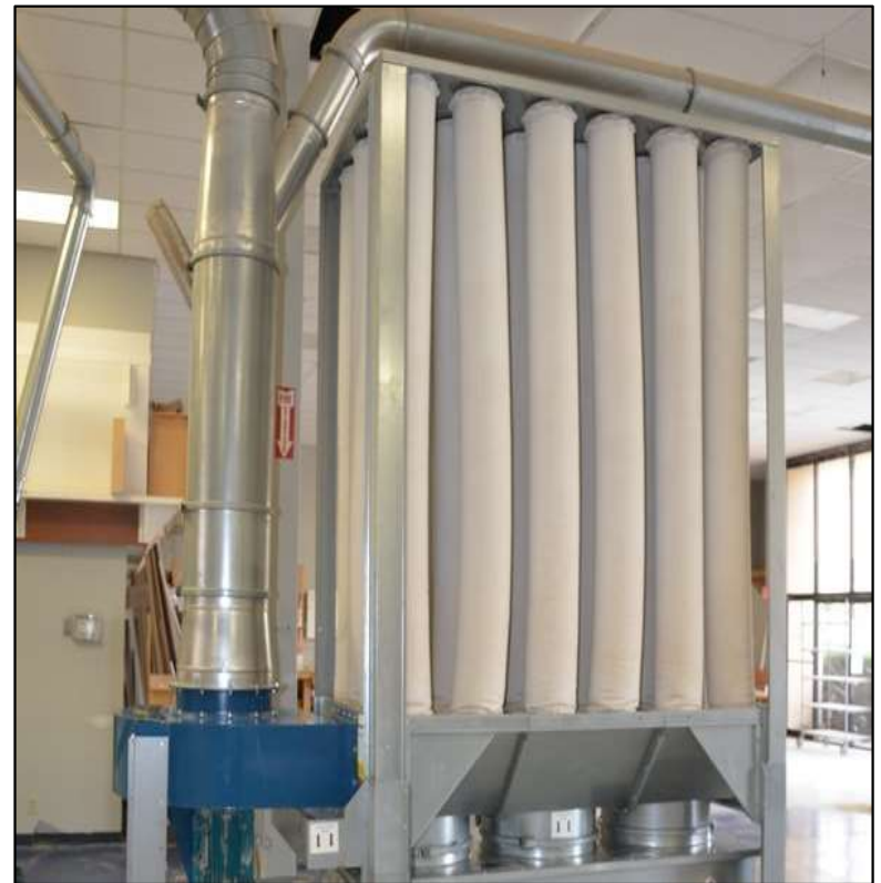
Example of a Small Open-sock Baghouse
