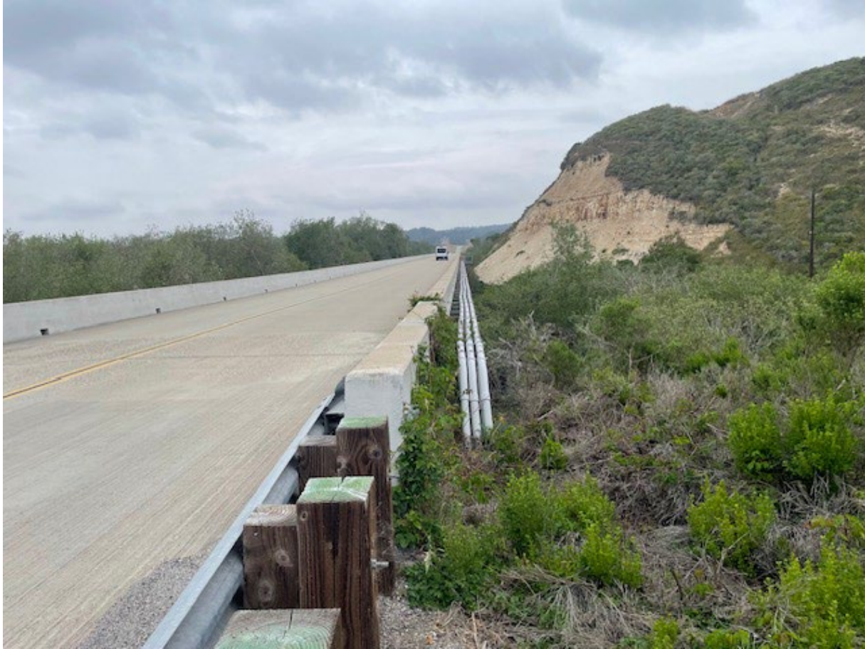
Figure 11. Close Up of Bridge Over El Rancho Pond
