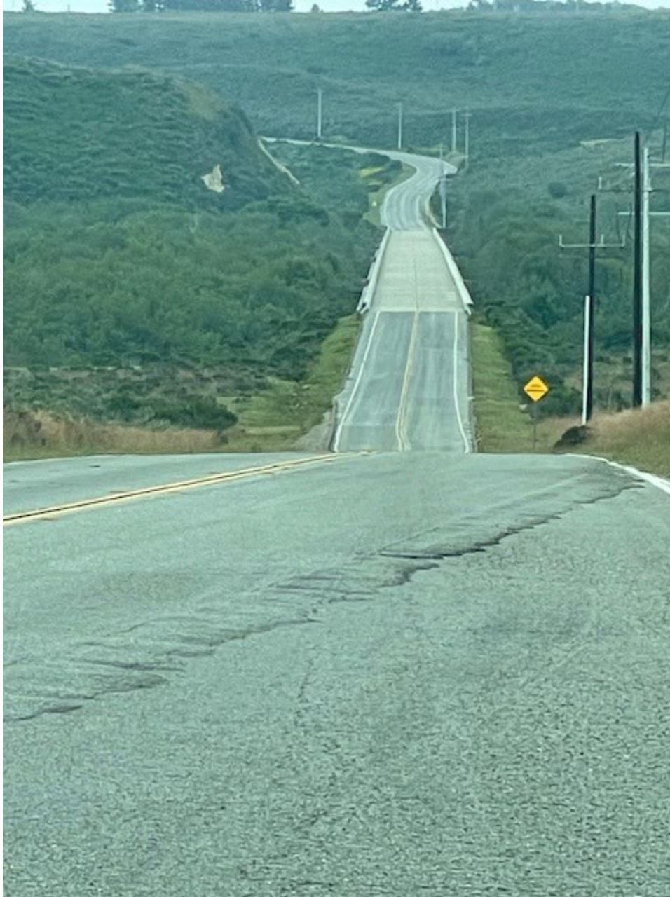
Figure 10. Bridge Over El Rancho Pond
